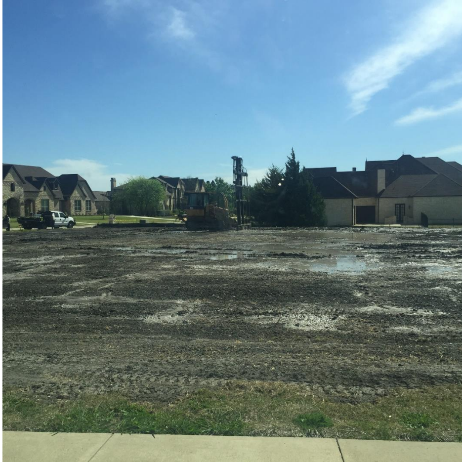
Chemical Application after Water injection
