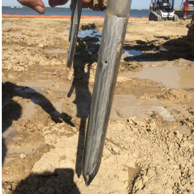
Steel Rod Holes for Chemical and Water Injection
